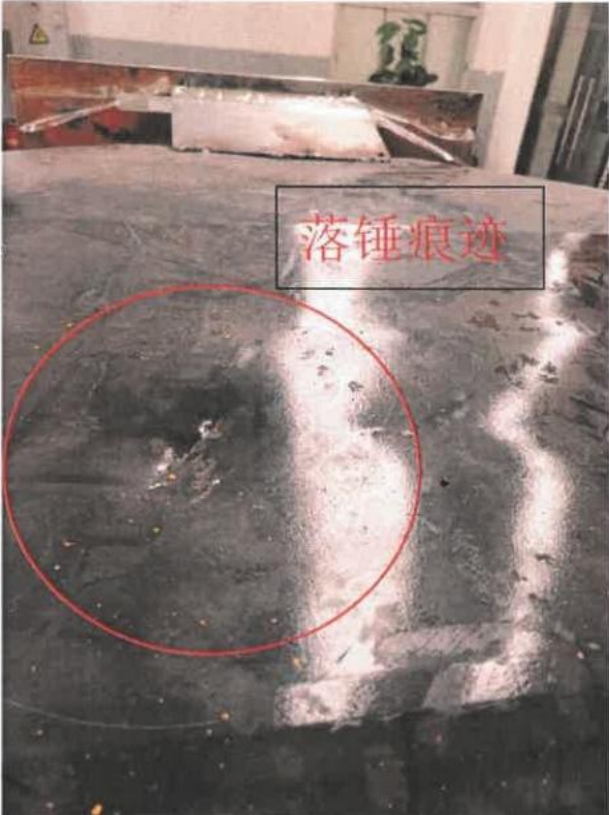
Photo F-1 hammer test
